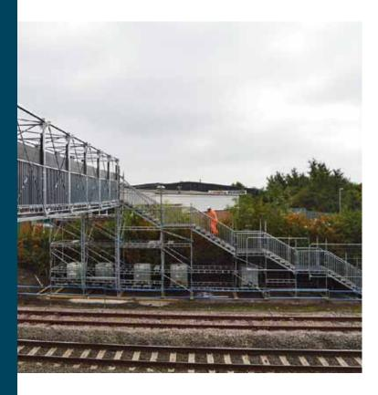
Stair towers provide a safe and quick access and egress to the workplace. The modular design and lighter components make the stairs quick and simple to erect.
